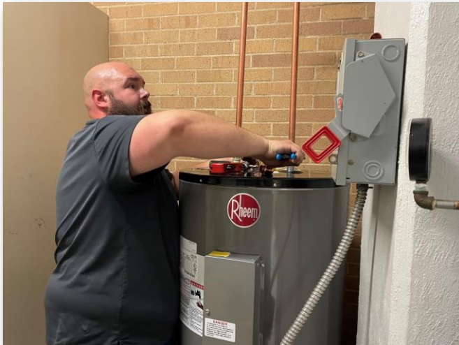
Ike in plumbing is finishing up a new water heater installation.
