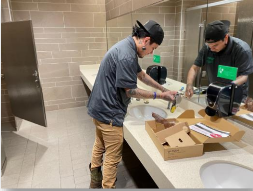
Nick in the plumbing shop replacing a sink faucet.
