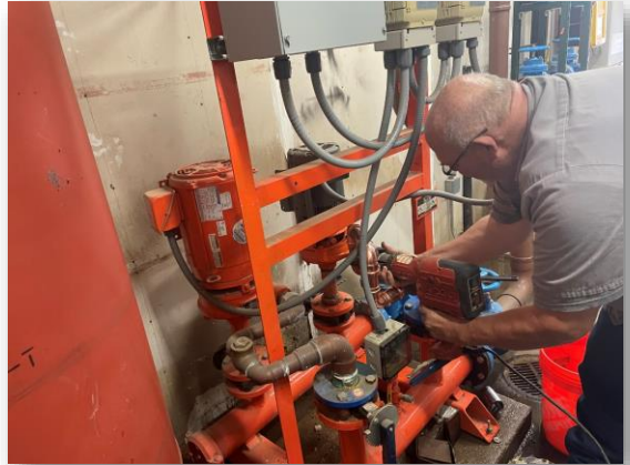
Bill Bullard repairing a leak on a domestic water booster pump.
