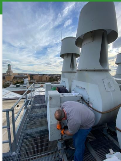
Mike and Clint replacing a bearing on an exhaust fan.
