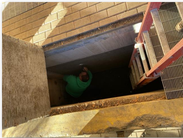
Eric from our Mechanical shop cleaning fresh air intake to ensure air quality in the buildings.
