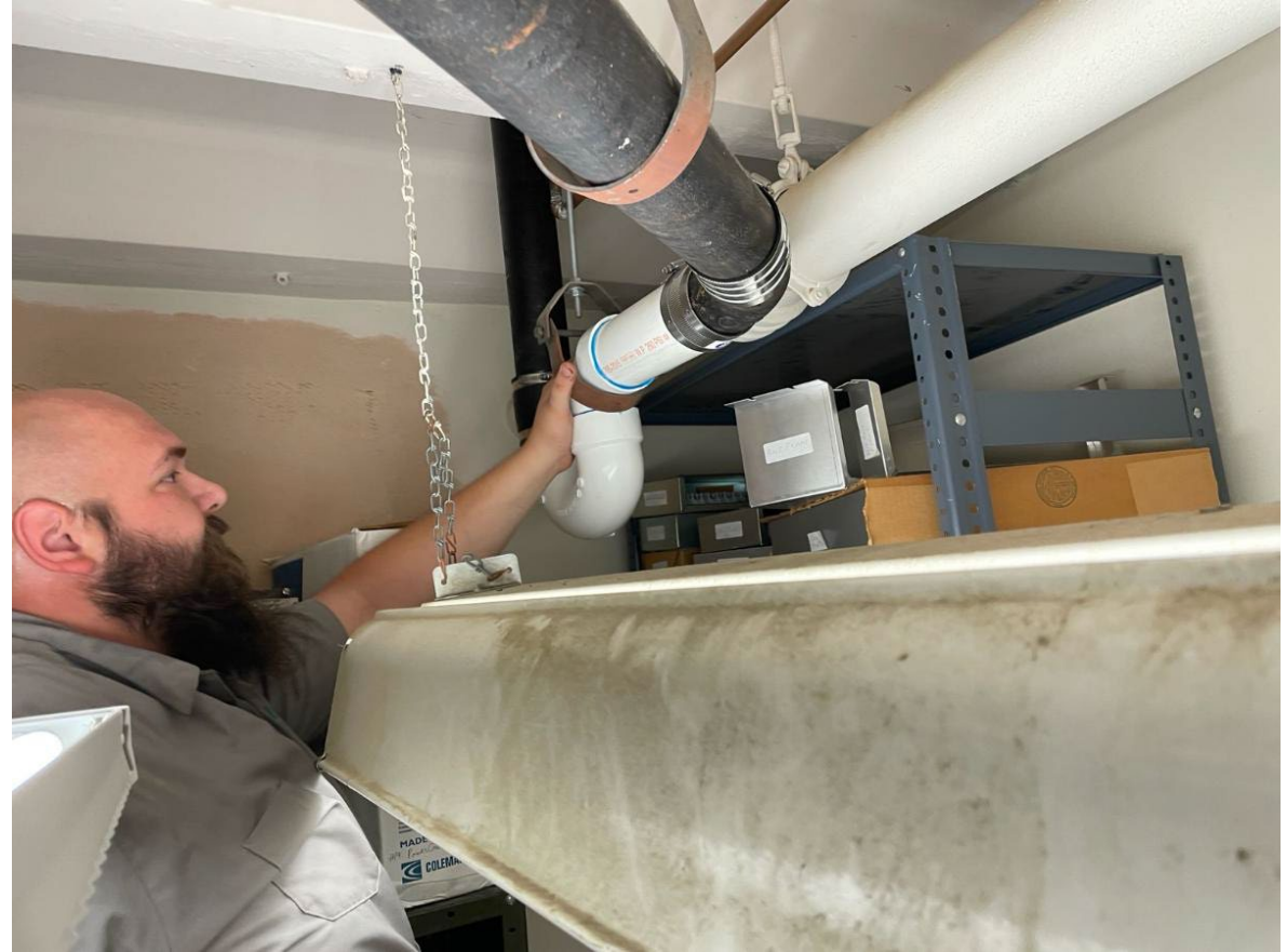
Ike replacing cast pipe with PVC
