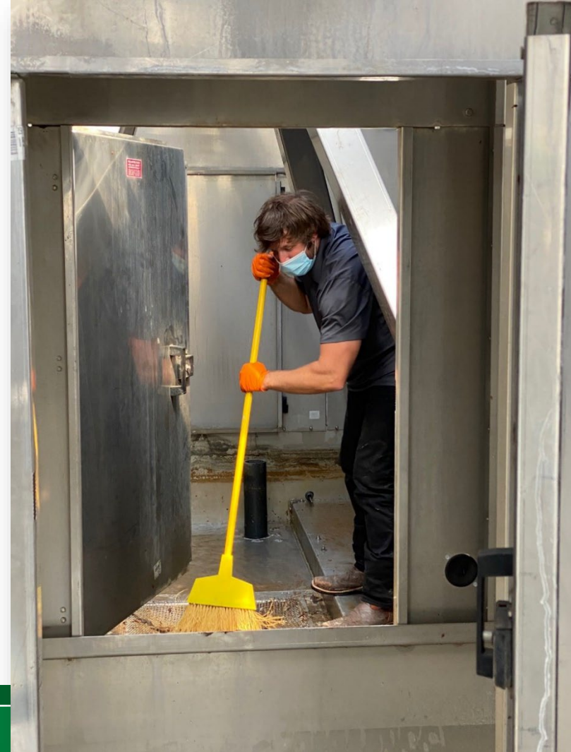
Adam cleaning a cooling tower
