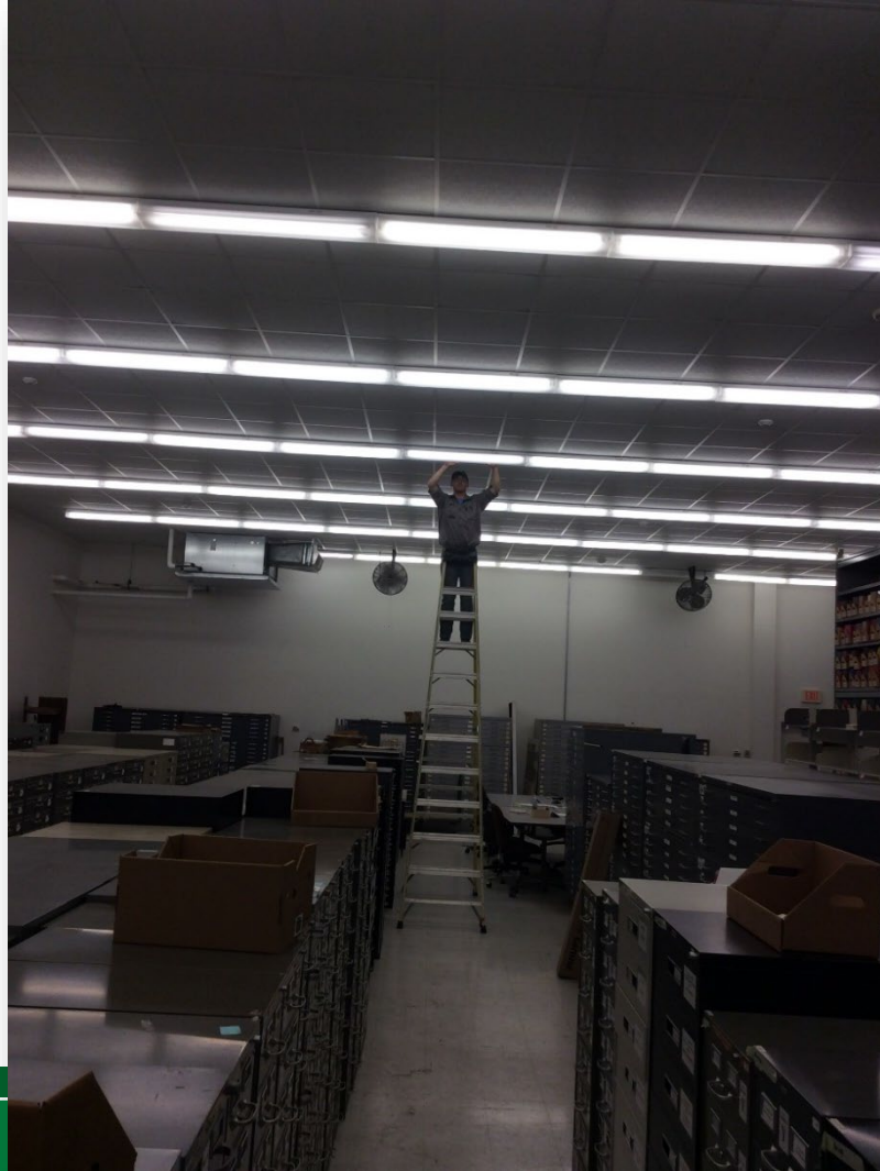
Technician on a 12' ladder replacing lights
