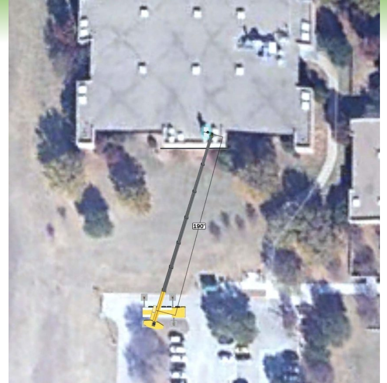
Crane Lift 7/30 south side of Wing E
