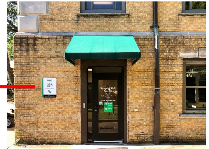
North East Corner of the building.
